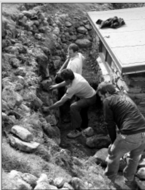
Mark, Alan and Jason rebuild the wall
